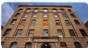
Police Station esquadra
