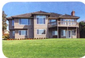
Detached house casa independente
